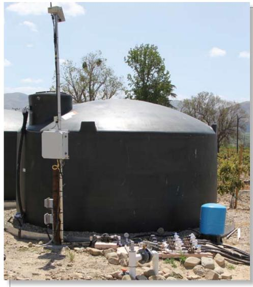
The water tank, irrigation controller, valves and flow meters used for the soil moisture sensor trial planting.
